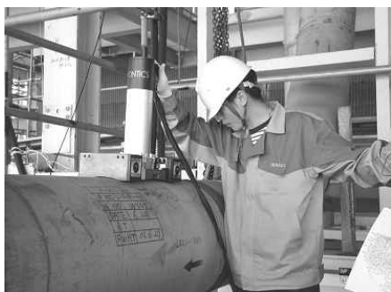
Photo 1 Residual stresses test for weldment of power plant main steam pipe
