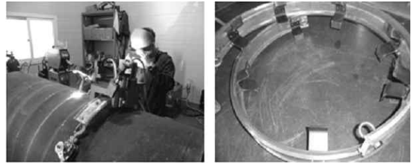
(a) Welding carriage (b) Pipe guide rail
