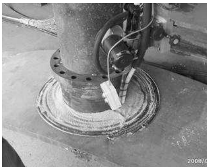
Fig. 5 Overlay welding for joining between nozzle to shell
