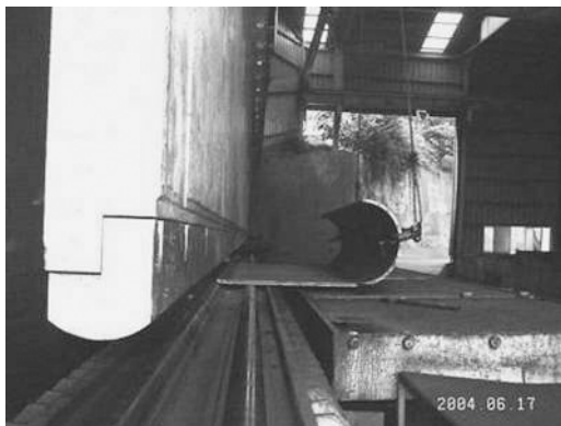
Fig. 1 Press bending of steel plate
