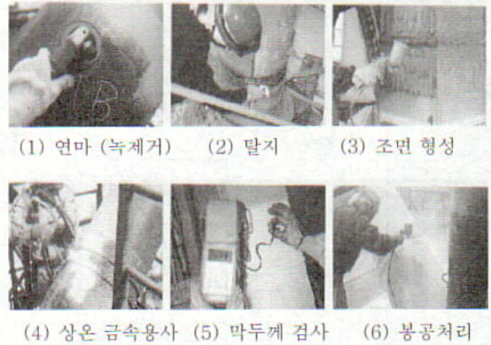
Fig. 2 Spray system Construction method of Zn·Al normal metal
