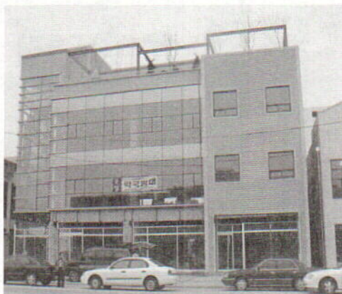
Fig. 6 Metal spray to steel wall Kangwondo, Gansung, 2002)
